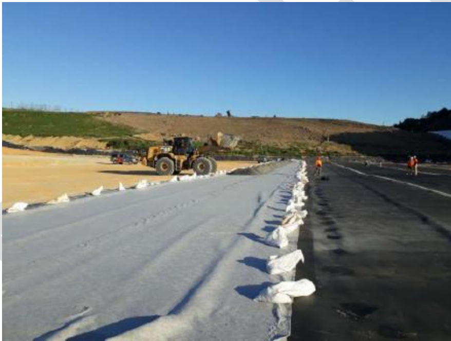
Figure 3d: Geotextile cushion and leachate drainage gravel
