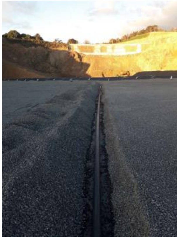
Figure 3e: Leachate pipe in leachate drainage blanket
